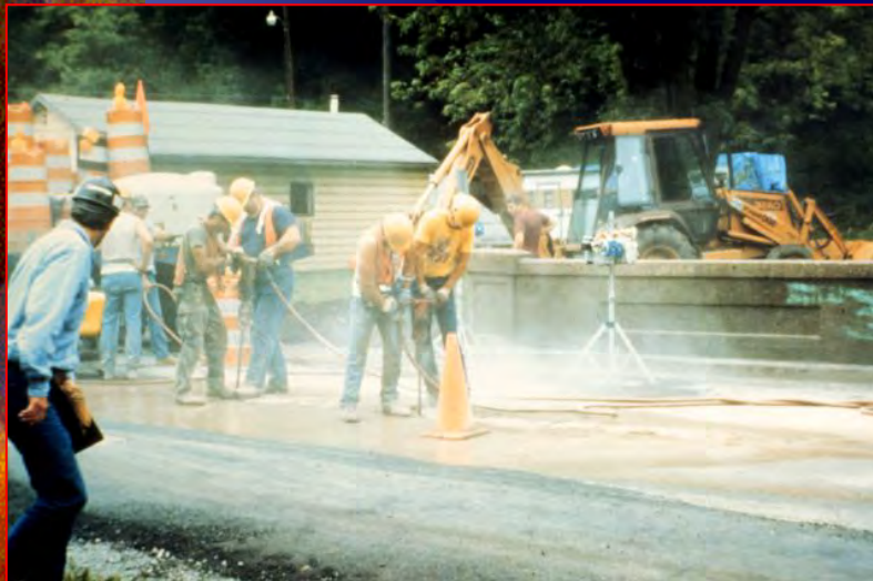
FIGURE 12. Jackhammer drilling without dust control. (About 1936.)
