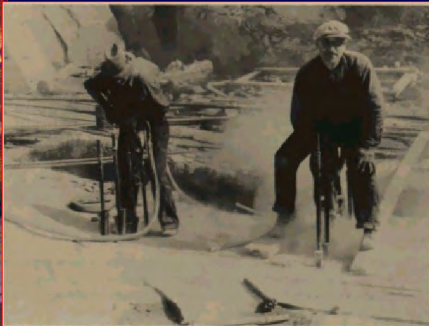
FIGURE 12. Jackhammer drilling without dust control. (About 1936.)
